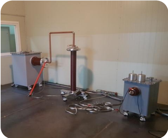
Partial Discharge Test
